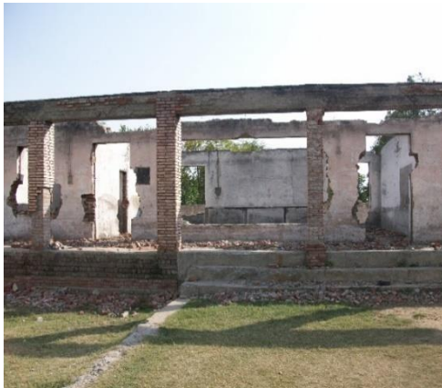
Figure 6. Condition of Wall-3
