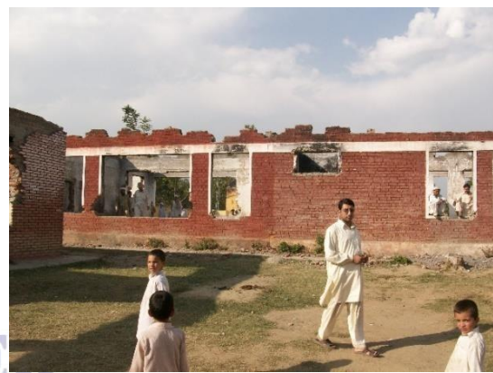
Figure 9. Condition of Wall-4
