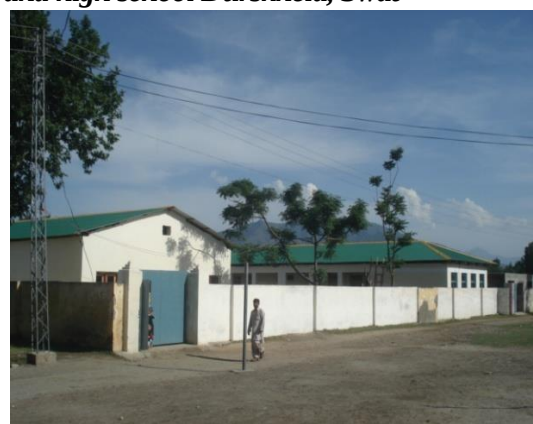
Figure 11. Condition of Internal Wall in Site
