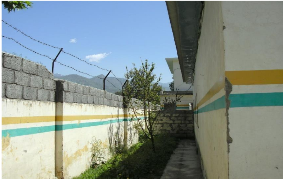
Figure 24. View form gate 2 of high school side wall.
