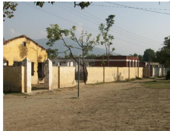
Figure 7. Condition of Wall-4
