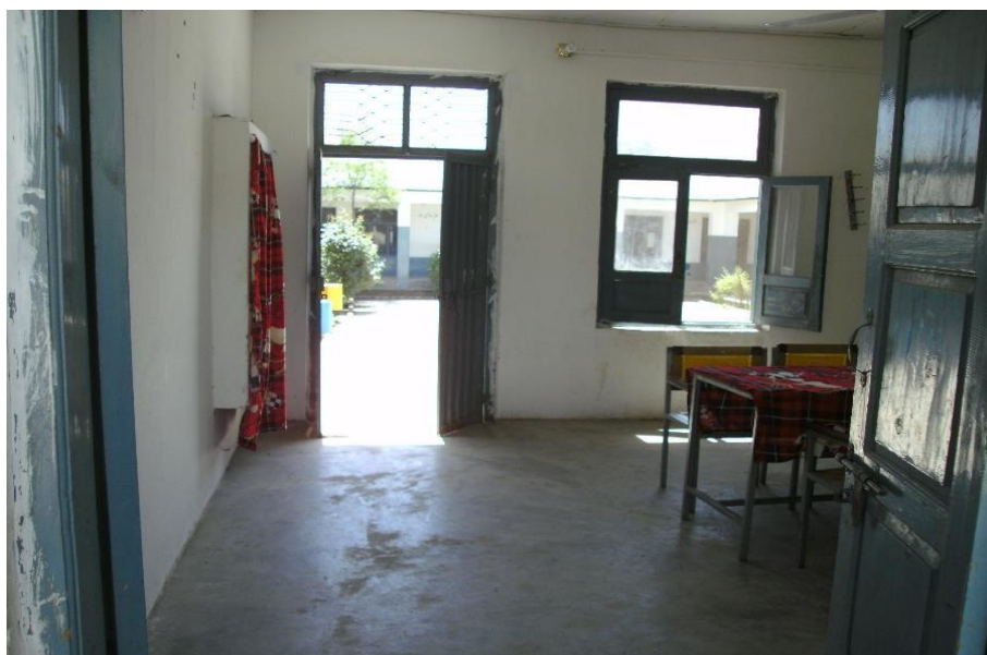
Figure 20. Visual from middle school staff room towards primary school courtyard
