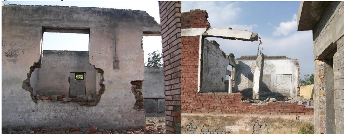
Figure 4 . Condition of Wall-1
