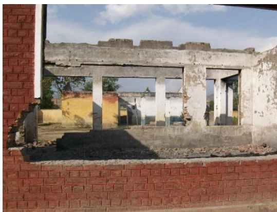
Figure 8. Condition of Wall-4
