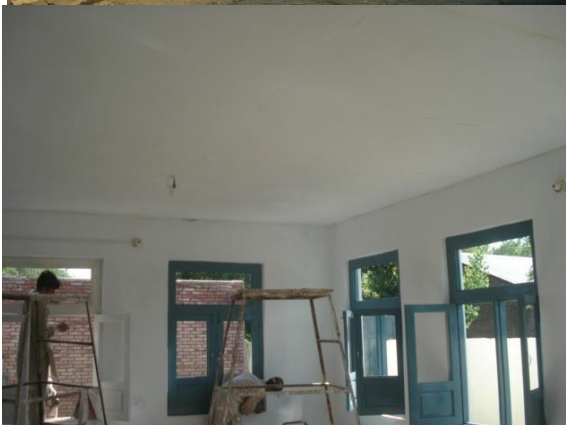
Figure 18.. Condition of Outer Structure Internal Walls
