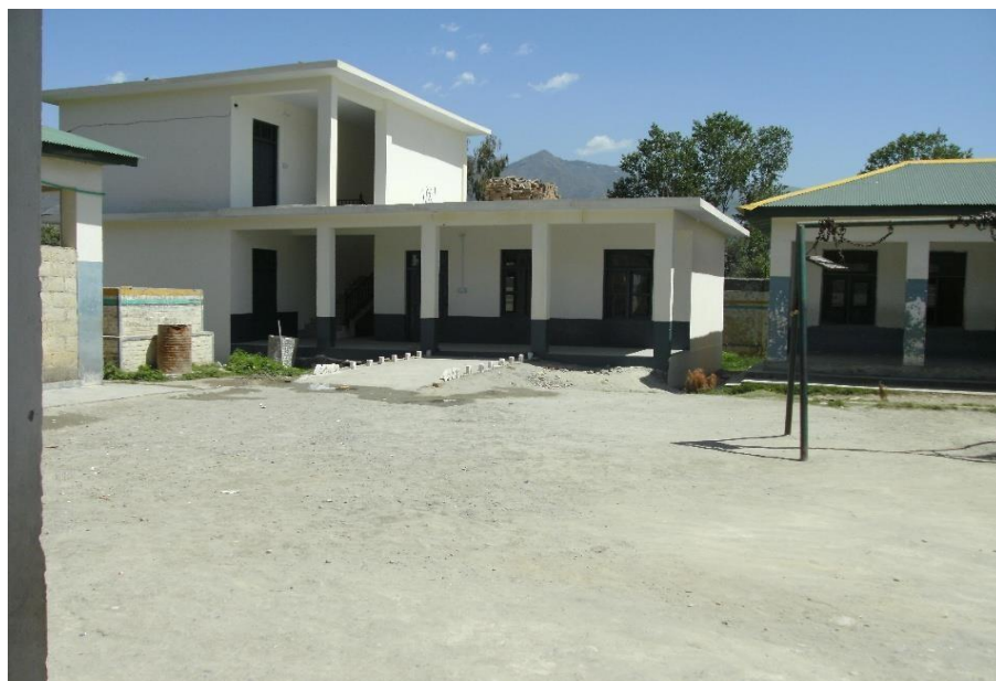
Figure 22. New constructed block for the extension of high school.
