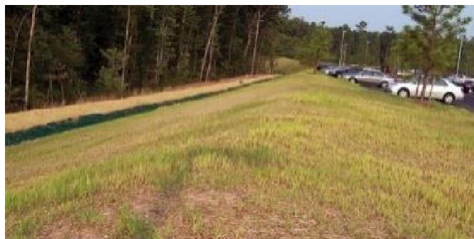
Figure 32 Uneven grading of site offers easy hiding places for criminals. Photo credit: Sean Ahrens.
