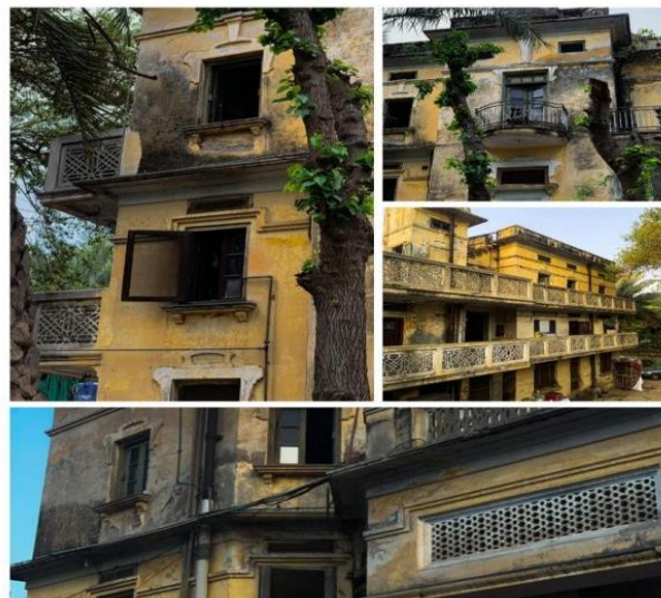
Figure 3: Deep overhangs and jali screens on the north façade, demonstrating principal shading and ventilation strategies.
