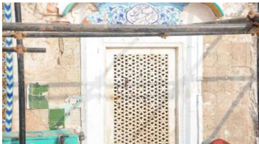
Picture 8: Lattice work on the south of the main chamber
