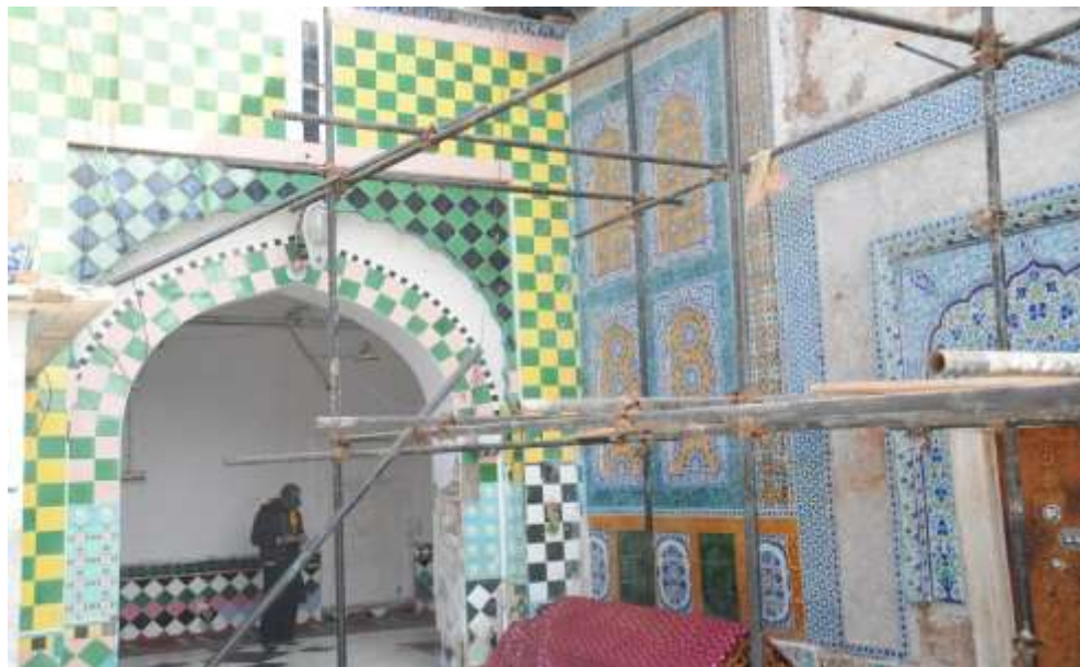
Picture 46: Restoration and renovation work at the shrine
