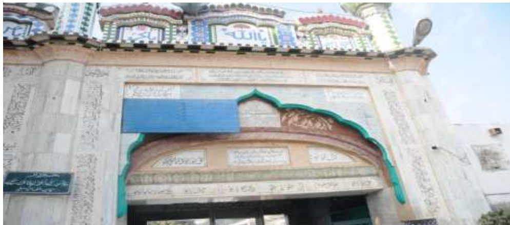
Plate 18: Front facade (darbar entrance)
