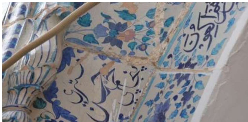
Picture 14: close up of the arch
