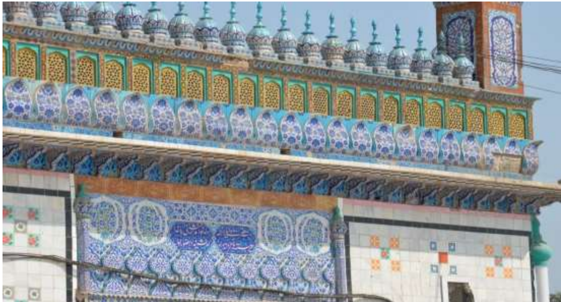
Picture 9: Blue tile work and lattice work on the parapets and frieze
