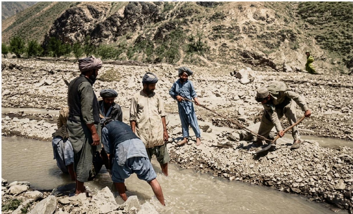
Pl. VIII- Constructing a traditional diversion weir somewhere in Balochistan (@ Oosterbaan, 1982).
